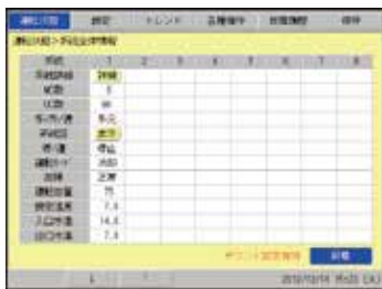
Operating Status/Main Screen
